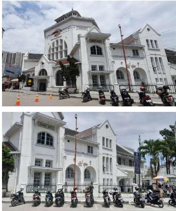
Gambar 4.96 Entrance Pos Bloc
