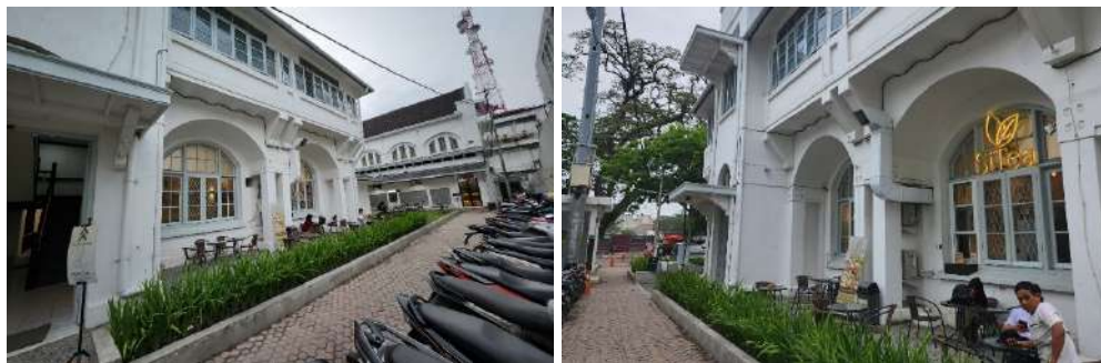
Gambar 4.97 Sisi Kiri Entrance Pos Bloc
